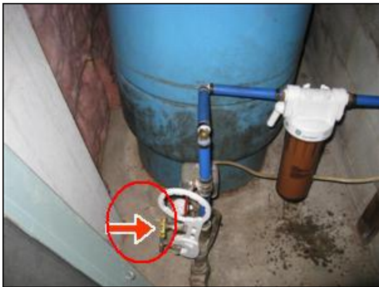
4.3 Picture 1 In basement
