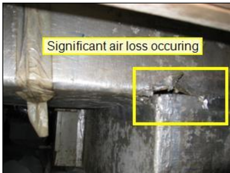
6.3 Picture 4 crawlspace new addition
