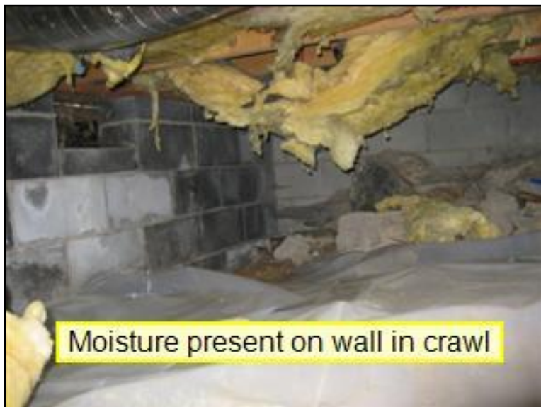
1.0 Picture 5 crawlspace under kitchen
