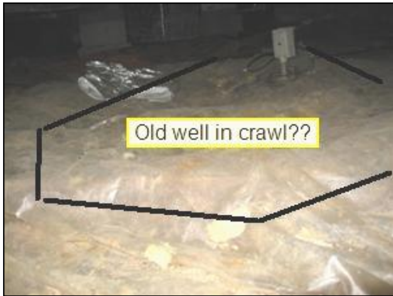
2.6 Picture 2 in crawlspace under new addition
